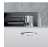
Installation on concrete
